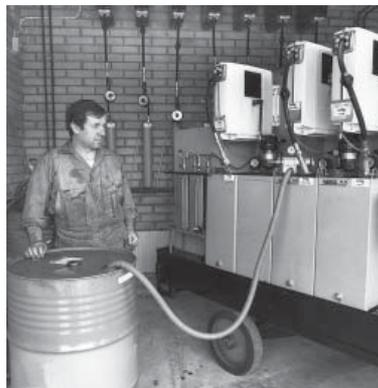
*It's simple to fill OriPac, because you only need one pump. No external pumps are necessary. OriPac makes it possible to store the lubrication oil in a separate oil store. The possibility to purchase larger quantities of oil gives better economy.*
